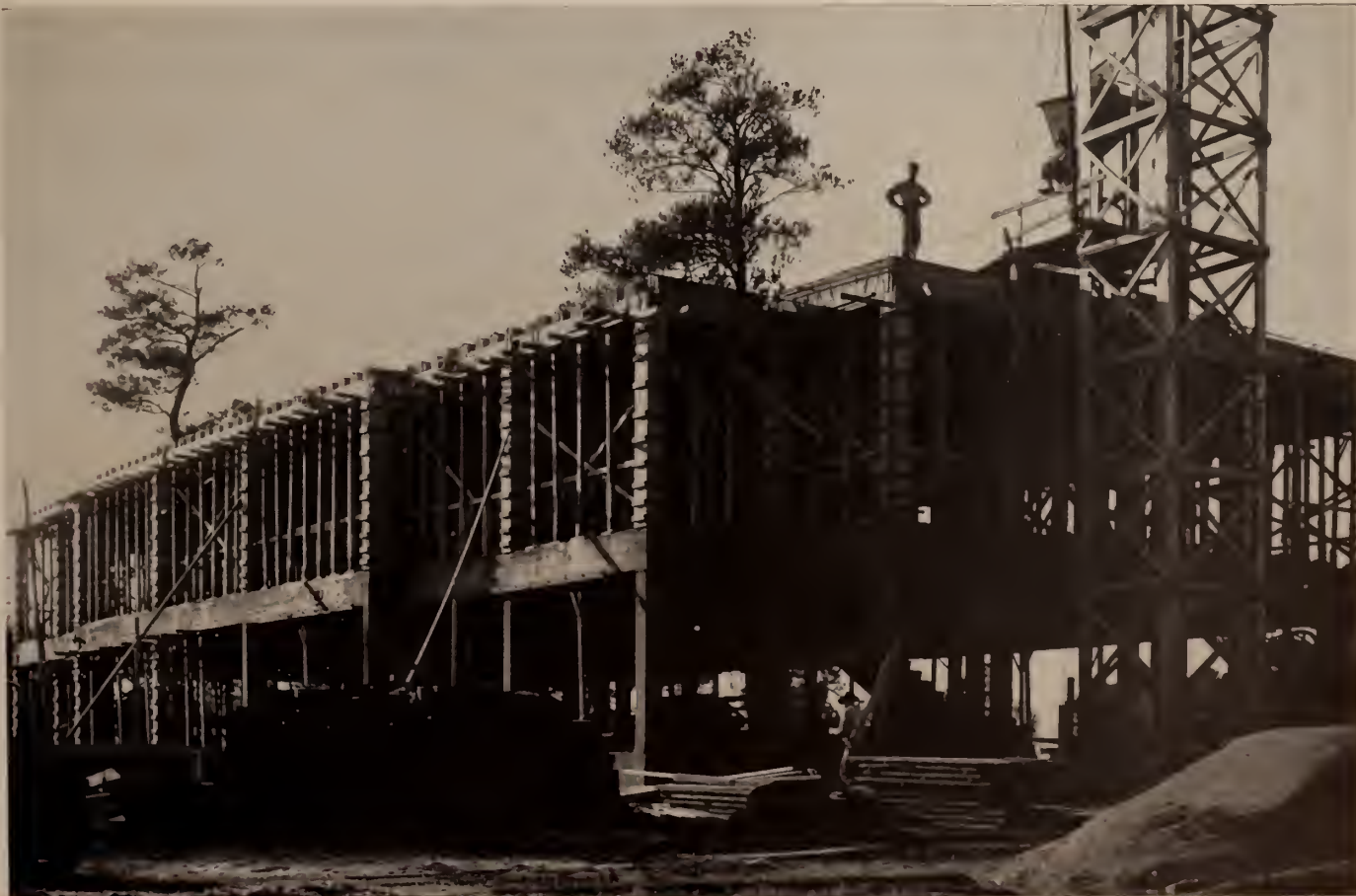
New Business Building under construction
